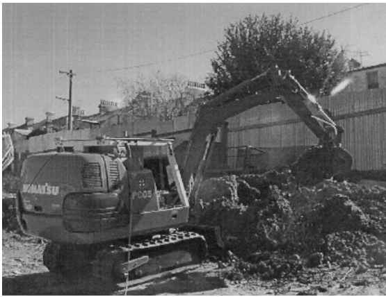
Fig. 3. Teleoperated robotic excavation.
