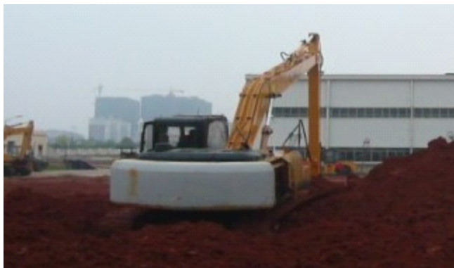
Figure 7. Digging test of excavator
